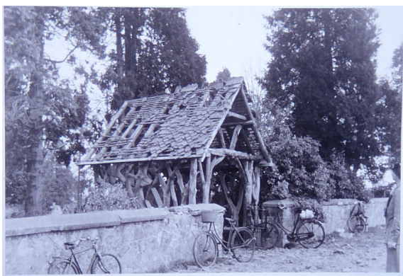
DAMAGE TO LYCH GATE
